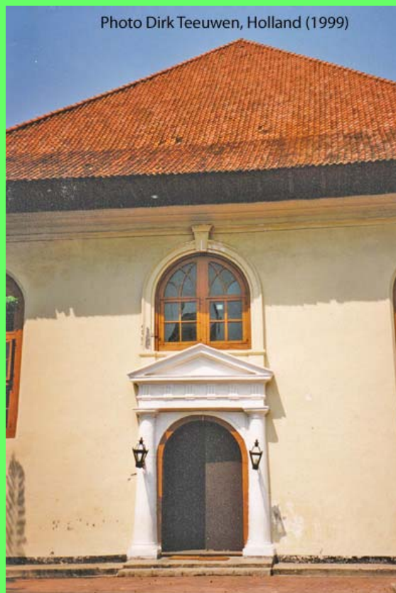
7. The northern entrance in close-up, 1999
