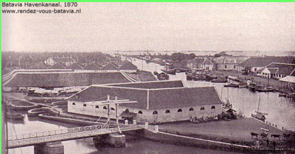
P. VI.7 Sunda Kelapa / Havenkanaal with Vierkants Bridge once again, Batavia 1870
