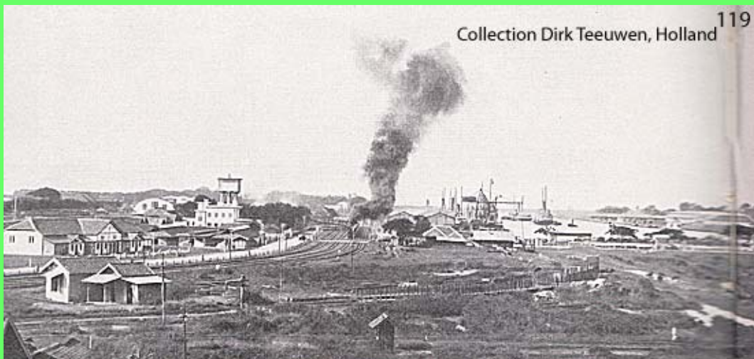
15 Tanjung Priok first harbour basin, 1927 View to the north, the wreath of smoke marks the location of the old (first) Tanjung Priok Railway Station.
