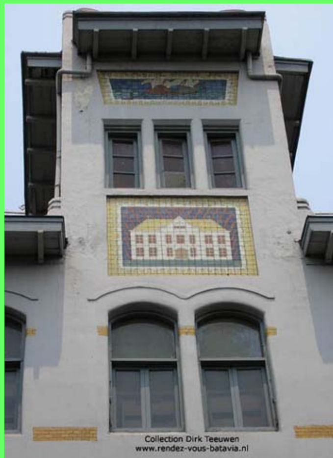
1.3 Detail of the copula tower of the former office of the Bataviasche Assurantie Maatschappij (Batavia Insurance Company). Kali Besar East 1996
