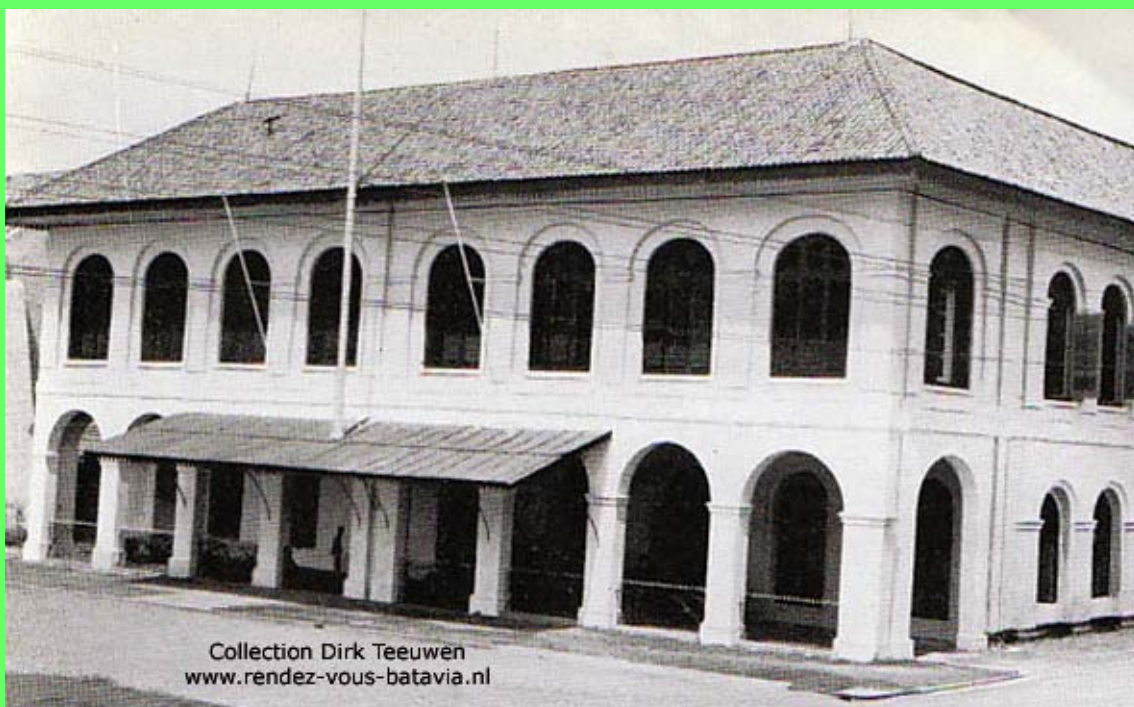
5.2 Office of McLaine, Watson and Company Import Export Insurance, northern end of Kali Besar West, 1936 (See p 4.6.)
