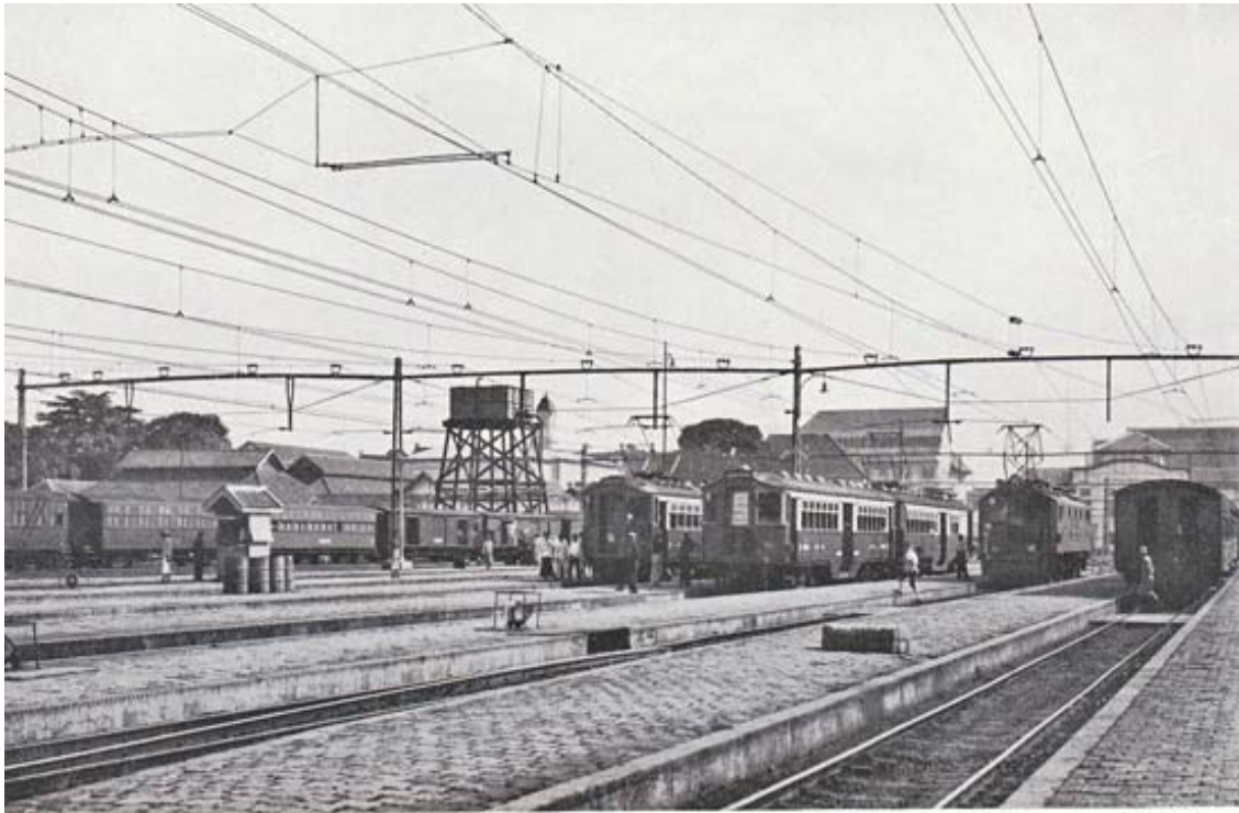
From "The importance of Java from the air" 1928 ARRANGEMENT OF THE OVERHEAD WIRES "SIEMENS SCHUCKERT SYSTEM" AT ONE OF THE STATIONS Collection Dirk Teeuwen, Holland
