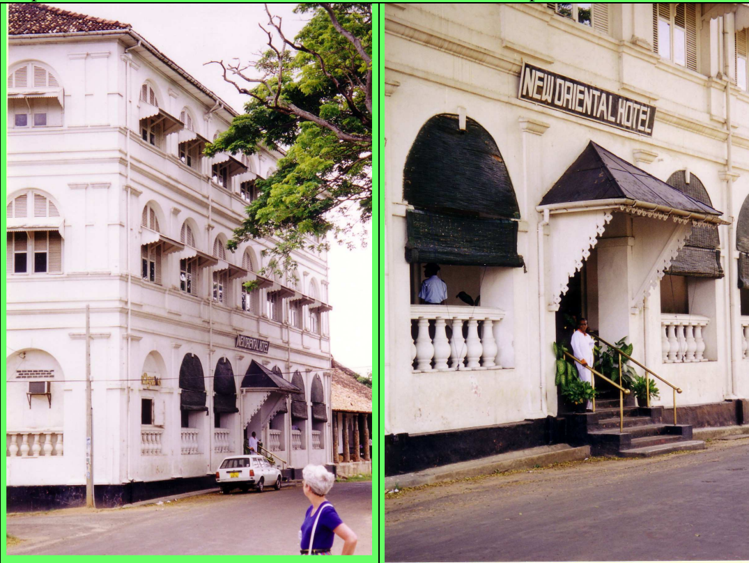
Afb. 1 Galle 1999, New Oriental Hotel from 1865 (1686 see summary), foto's Dirk Teeuwen (DT) At the right side of the hotel one can see a part of V.O.C.-commander's residence. The residence is now Dutch Period Museum.
