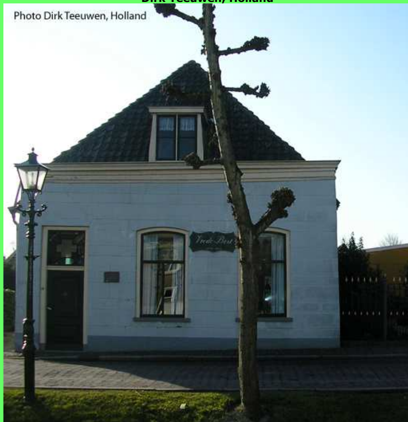
A farmhouse, from 1783, built within the town ramparts; Nieuwpoort 2015
