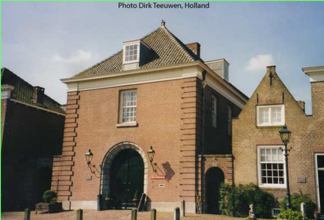
The armoury, built in 1781; Nieuwpoort 2014
