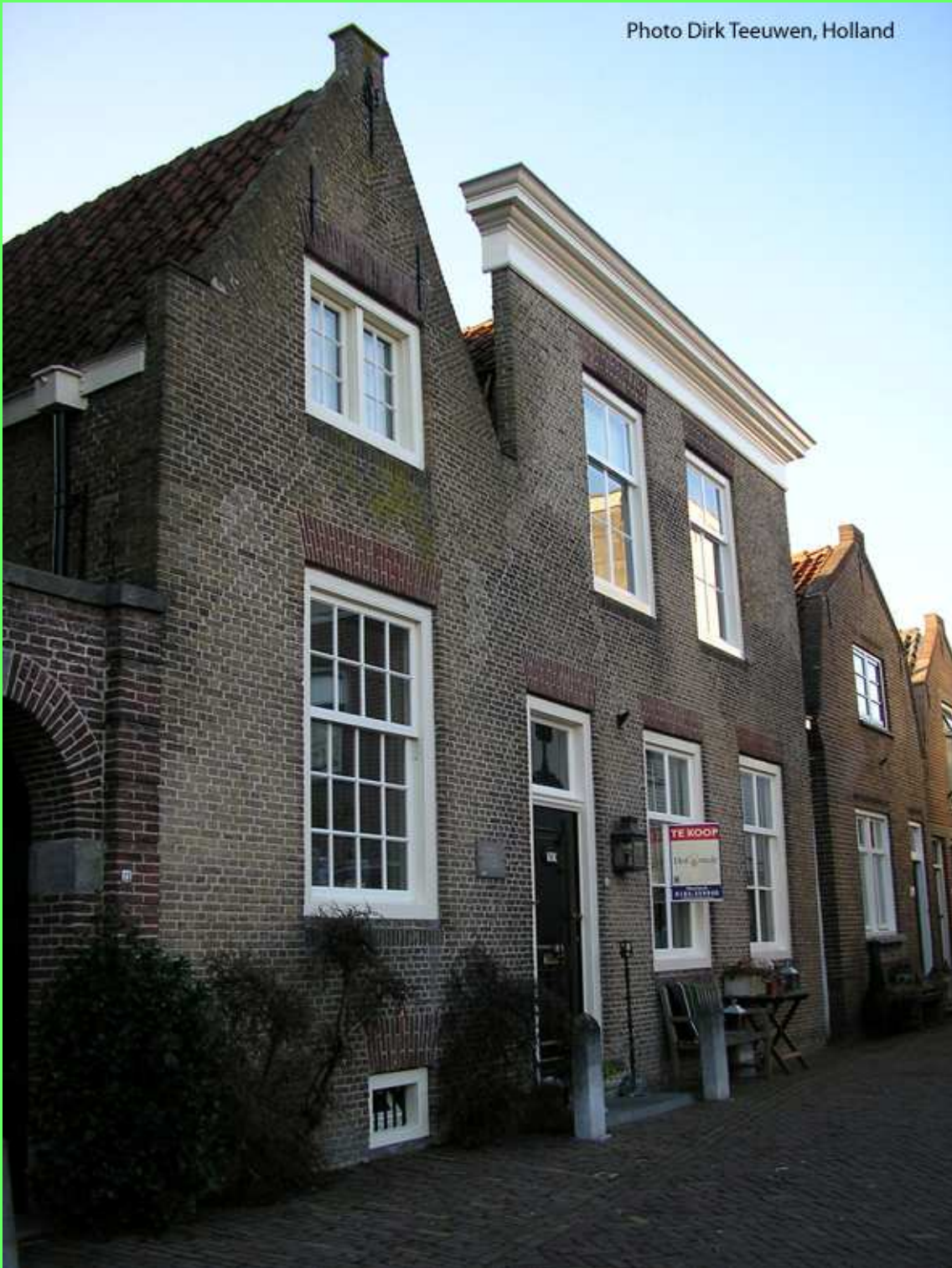
House of the bailiff (left), built 1570; Nieuwpoort 2015-02-17
