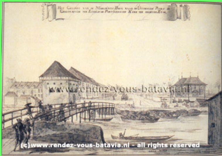
Picture 8. The Portuguese Church inside the Walls in 1776, drawing by J. Rach. View from the New Mint-Bridge / Nieuwe Muntbrug (crossing Kali Besar) to the west. Across the bridge, in front of us, we look into Jn Kopi / Utrechtse Straat, the Utrecht-Gate / Utrechtsche Poort and the Portuguese Church at the right behind a brick cemetery-wall..
