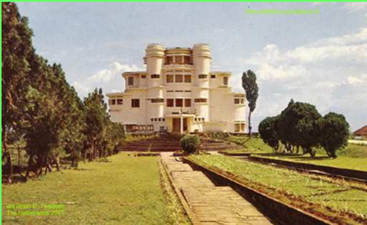
Picture 1. Villa Isola,northern façade, Bandung 1956
