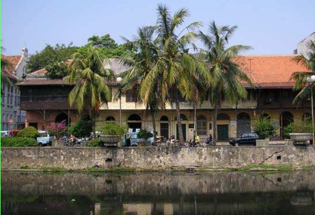
5 Kali Besar Timur, 19 th century offices
