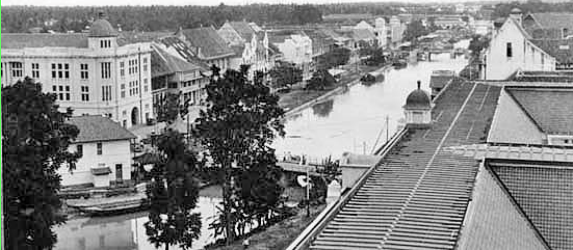
2 Southern side of Jakarta's Kali Besar Barat, 1930
