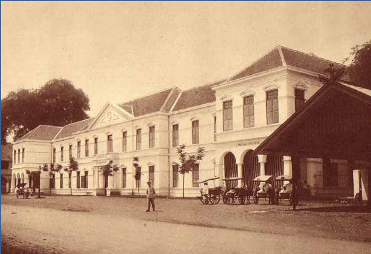
P.19 Military hospital in Jakarta / Batavia near Jl Kwini 1 / Mendjanganweg, 1926 In the 17 th and 18 th century this was the location of the country estate "Weltevreden".
