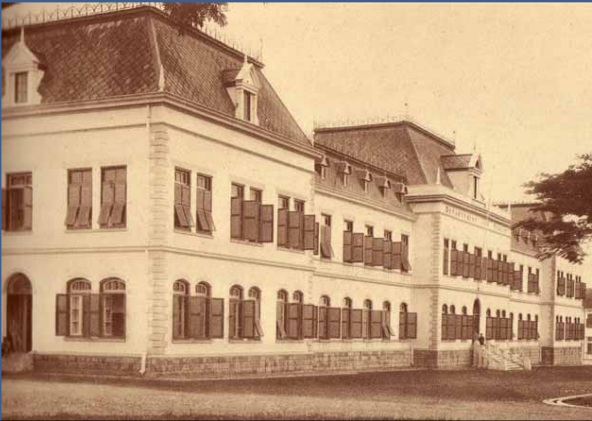
P.2 The office of colonial department of war, Taman Lalulintas / Insulindepark in Bandung / Bandoeng 1926. The department was subordinate to the Ministry of Colonial Affairs in The Hague. Before 1915 the offices on P.2 and P.3 were located in Jakarta / Batavia
