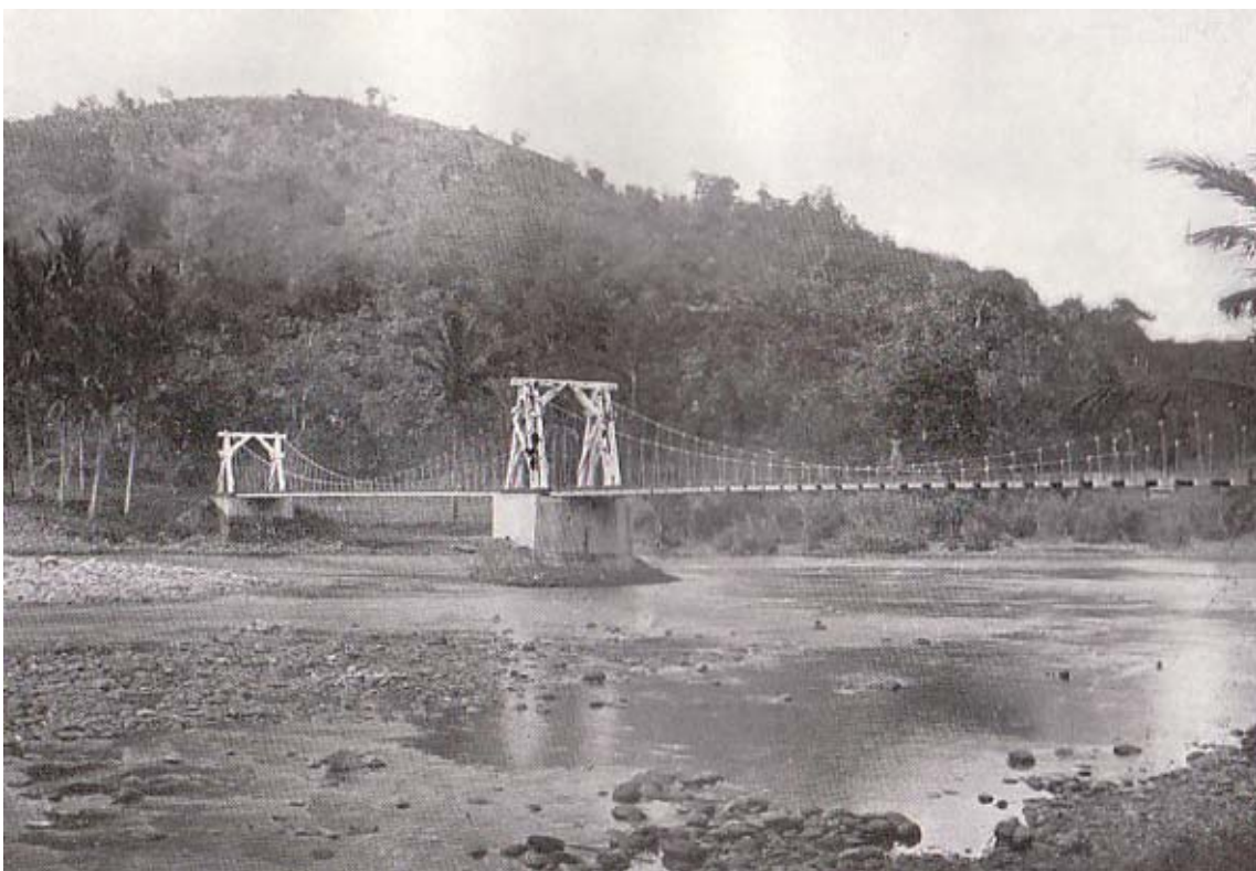
Cable bridge across Lematang River near Pulu Pinang, 1911
